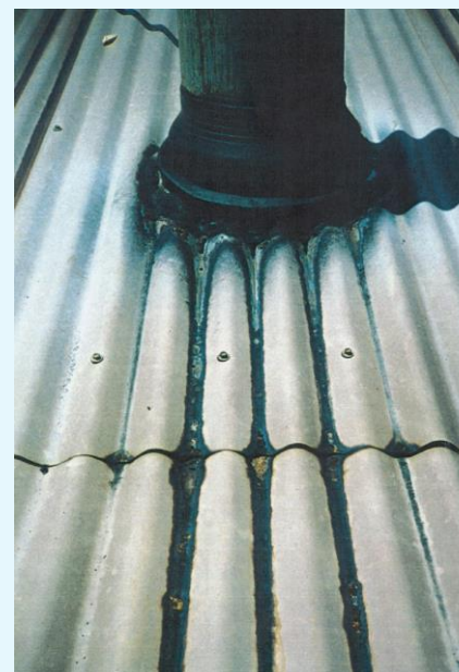
Figure 1: Flue Deposition/Corrosion.
